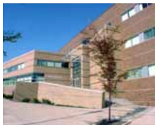
Rutgers Public Safety Building New Brunswick, NJ
